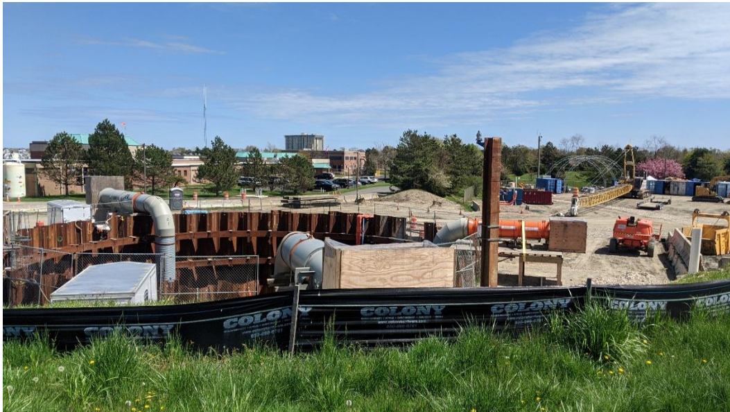
Excavation for the New Main Pump Station at the TRWRA Plant in Monmouth Beach
